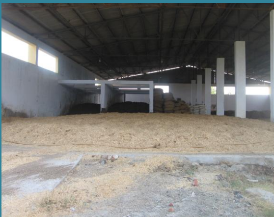
Fig.2: Composting yard including Phase-I bunker Bunker
